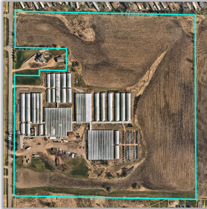
Figure 1 Project Site 7600 Maple Hill Road
