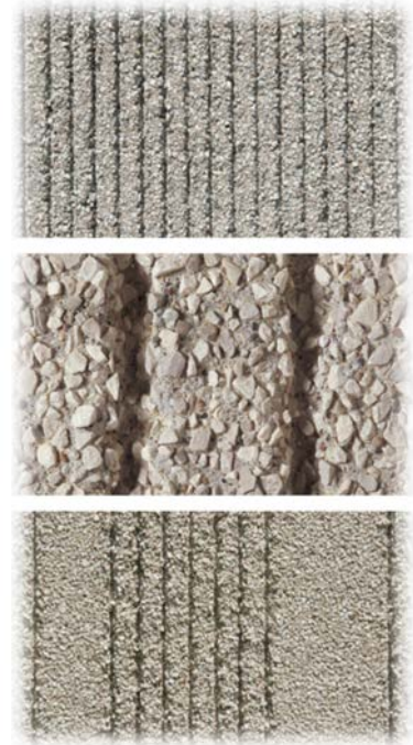
Ribbed Precast Concrete Panels
