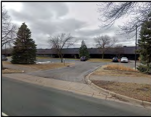
Maple Grove office / warehouse 02 front
