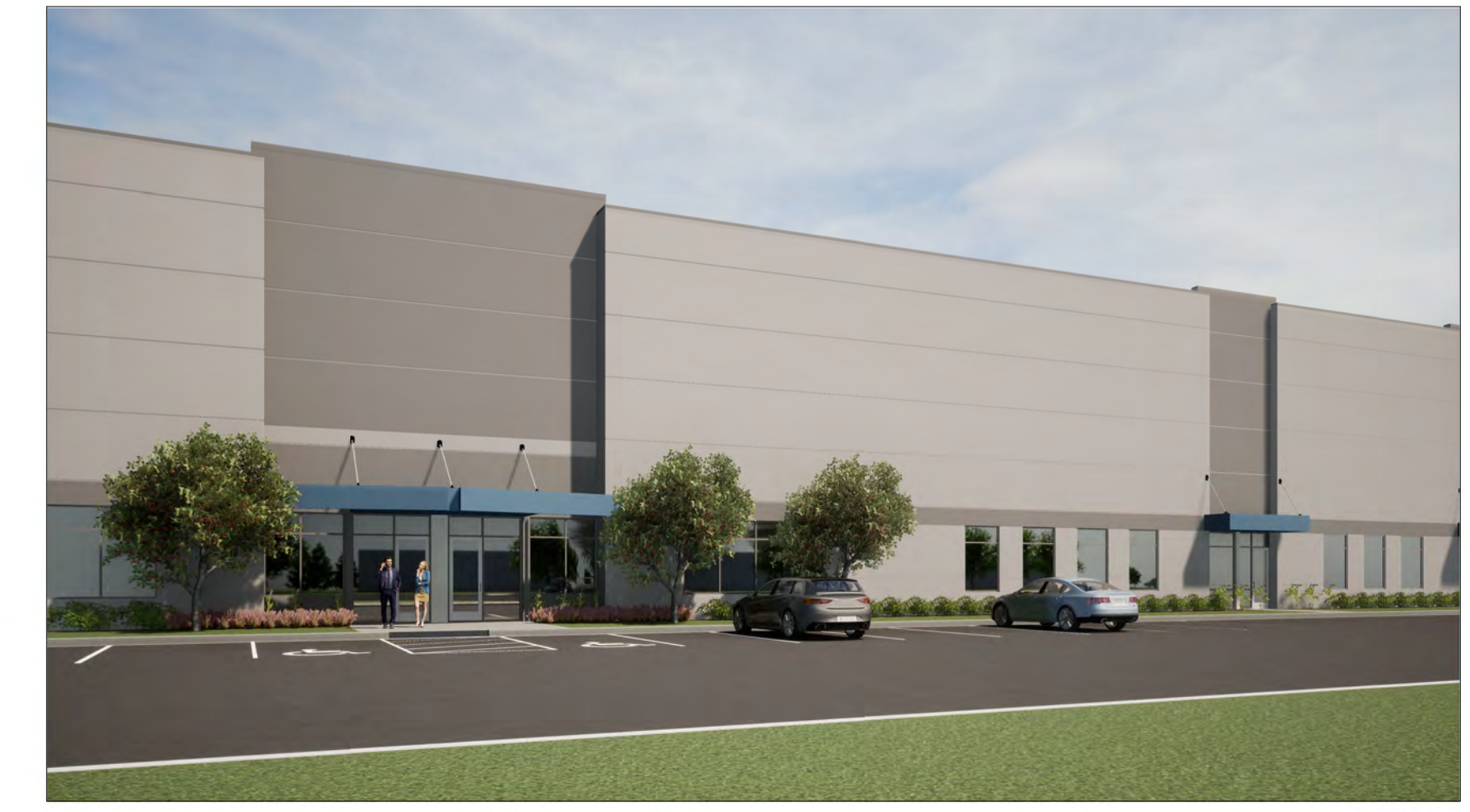
VIEW 2 - BUILDING C NORTHEAST CORNER
