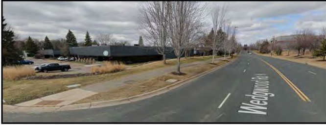
Maple Grove office / warehouse 01
