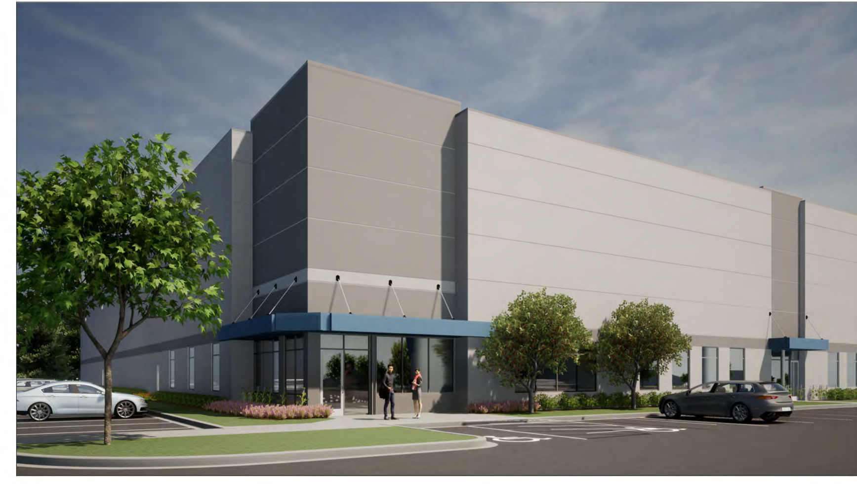
VIEW 1 - BUILDING C TENANT ENTRY
