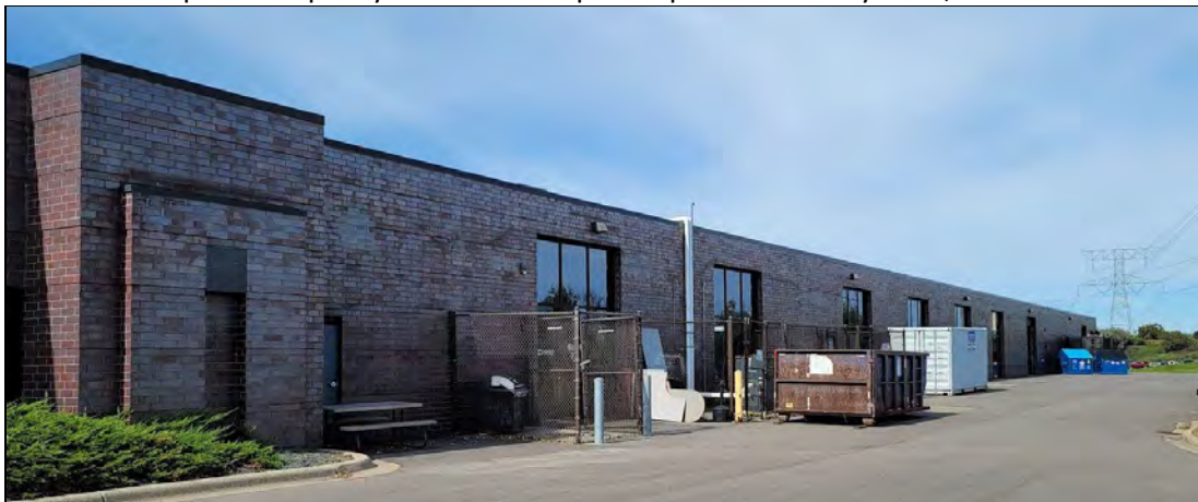
BACKSIDE OF MAPLE GROVE WAREHOUSE
